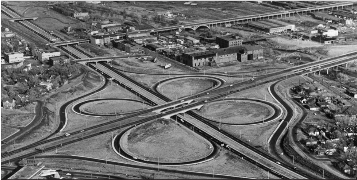
New highways built under the National Interstate and Defense Highways Act standardized lane and shoulder widths, underpass heights, and the frequency of exits. This photograph shows a newly completed cloverleaf interchange in Denver, Colorado, in 1958.
