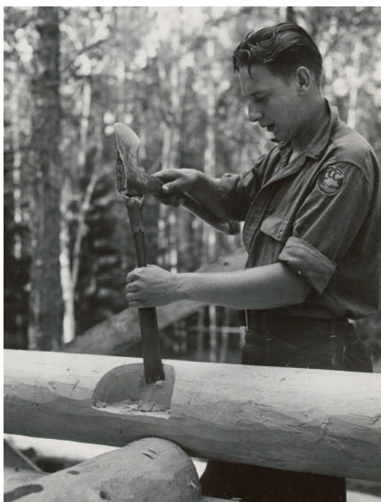
CCC worker Leslie Anderson cuts a notch out of a log that would be part of the new LaCroix Guard Station in Superior National Forest.
