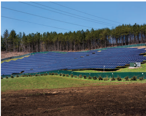
In Murphy, North Carolina, solar panels generate electricity directly from sunlight.
