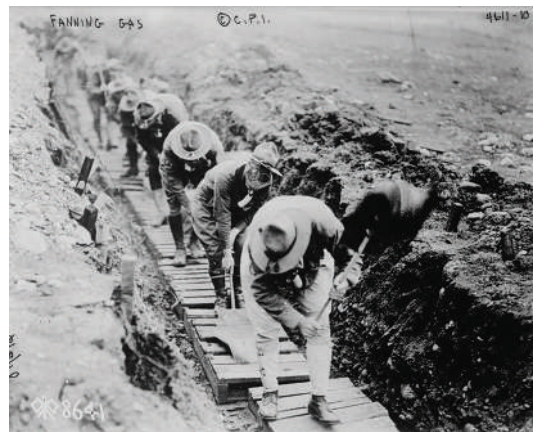
At Camp Kearny, north of San Diego, soldiers learned many things, including how to use a trench fan to clear poisonous gases.
