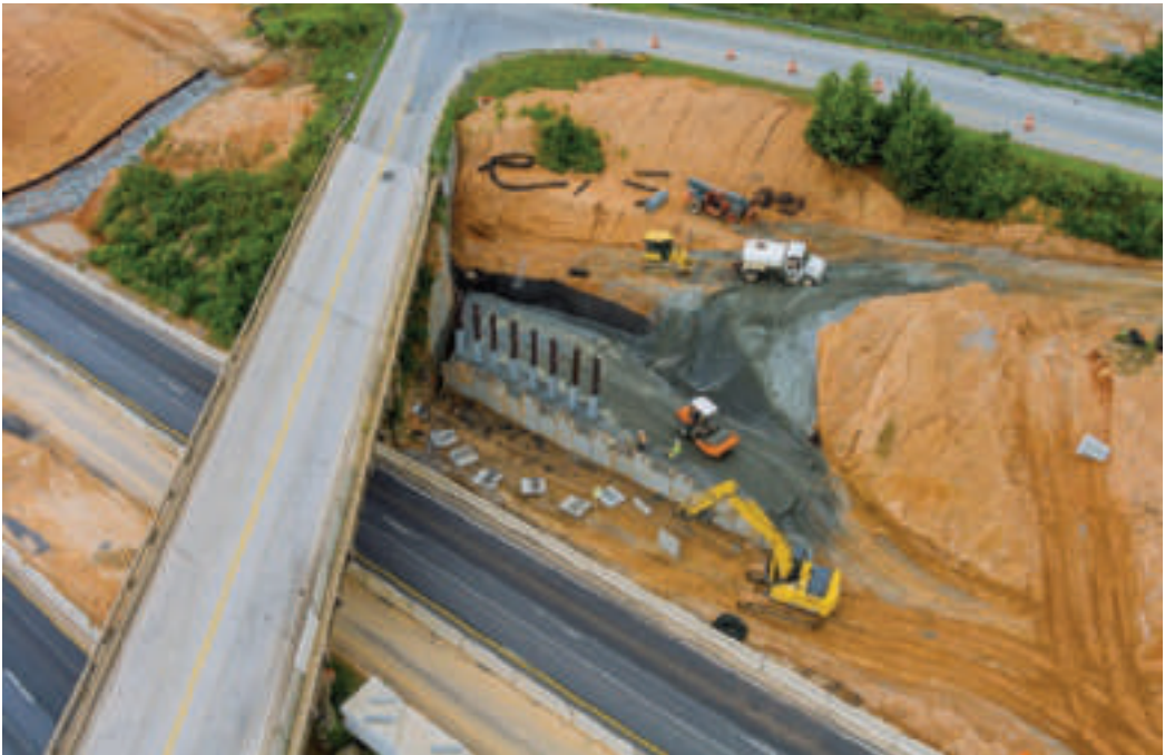
States work with the federal government on major highway construction.
