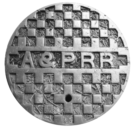
Utility Hole Cover
