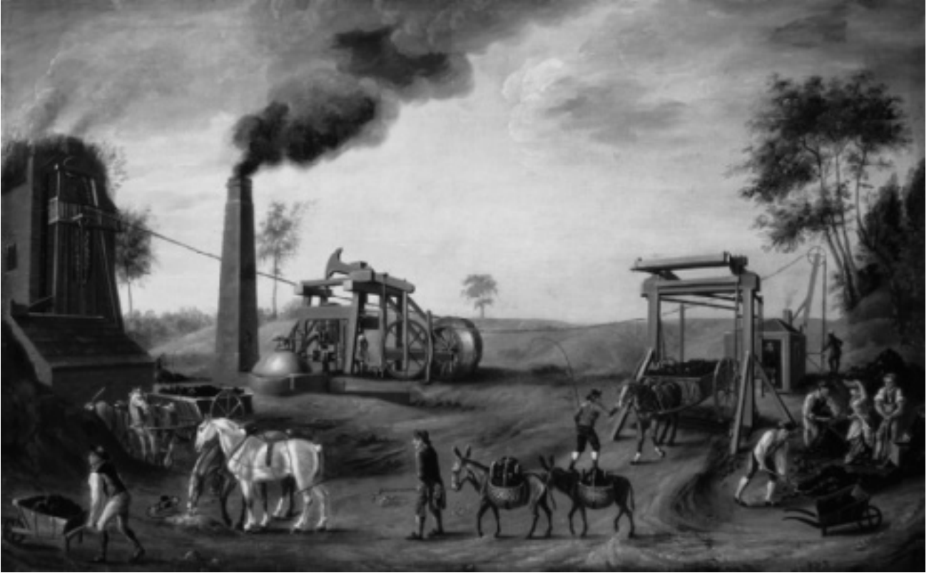
The steam engine pumped water out of coal mines, making it easier, safer, and quicker to dig for coal.
