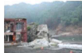
Close-up of the broken seawall after the 2011 tsunami.
