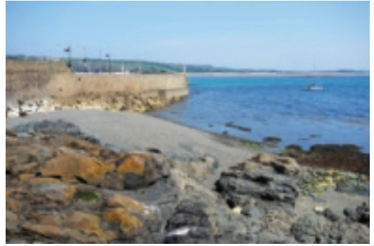
An example of a vertical seawall.
