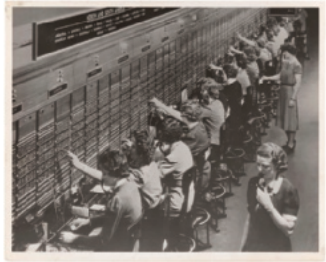
Telephone switch operators.
