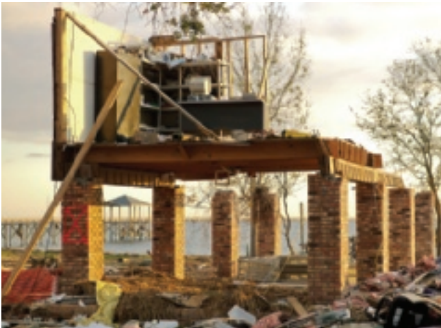
These brick-and-mortar piers serve as ruins for the structures that survived Katrina's wind and storm surge. The wood-framed house perched above was destroyed. Somehow the computer did not budge from the desktop.
