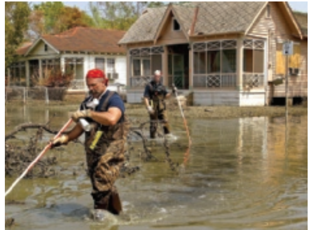
These homes in New Orleans withstood the winds, but the severe flooding means they are most likely uninhabitable due to wood rot, mold, and bacterial growth.
