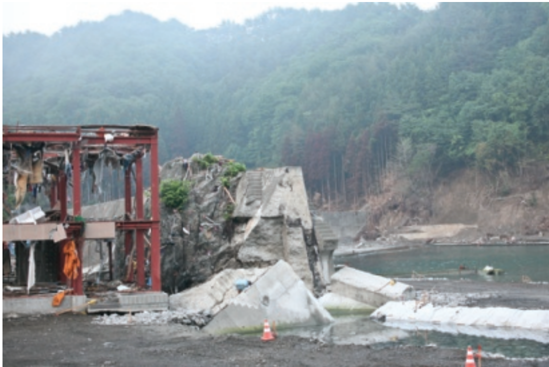
Close-up of the broken seawall after the 2011 tsunami.
