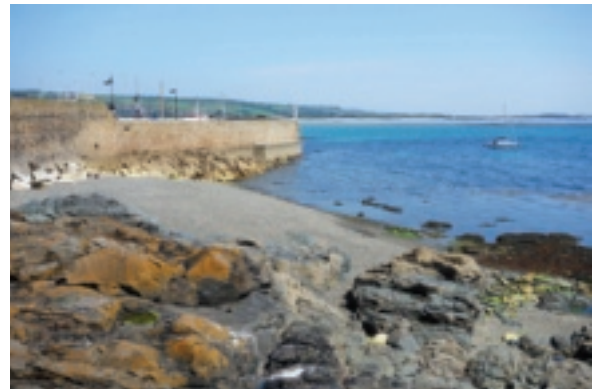
An example of a vertical seawall.
